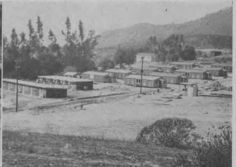
FPHA project on Raley Drive
