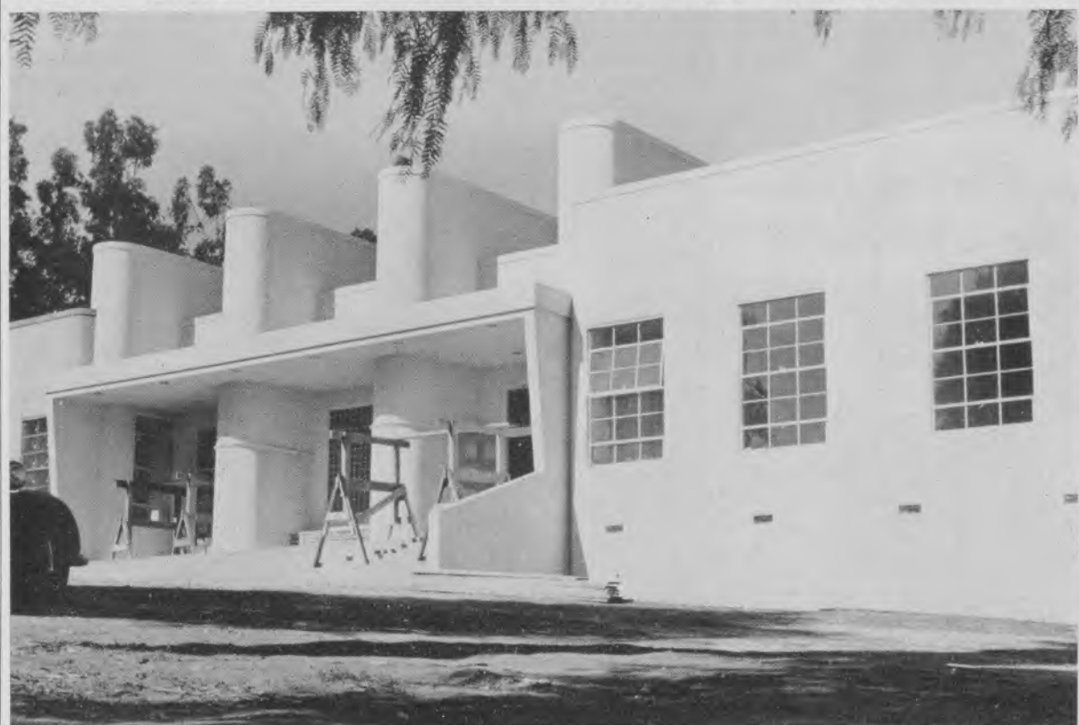
Latest addition to La Sierra college campus is the gleaming white science building, shown above. Rapidly nearing completion, the structure will house the Biology and Chemistry departments. Present plans call for occupancy in early summer, according to W. E. Anderson, LSC's business manager. Cost of the building, minus scientific equipment, is $160,000.
