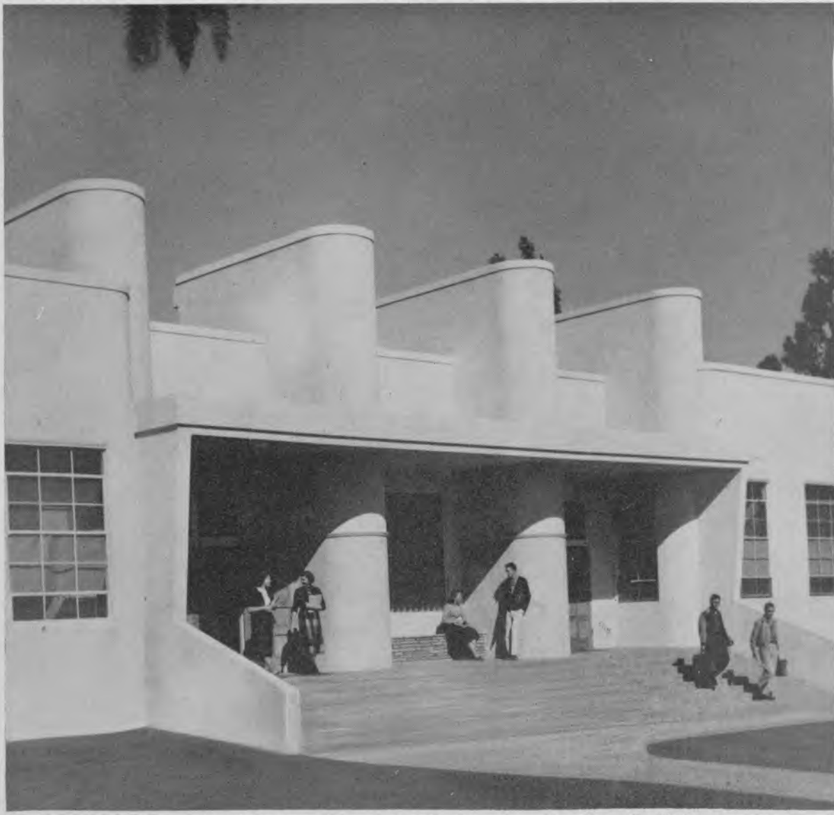
PALMER HALL in which a number of improvements have been made during the past summer. Specifically, a concrete floor in the basement of the Biology department, a water distilling unit for the Chemistry department and cabinets.
