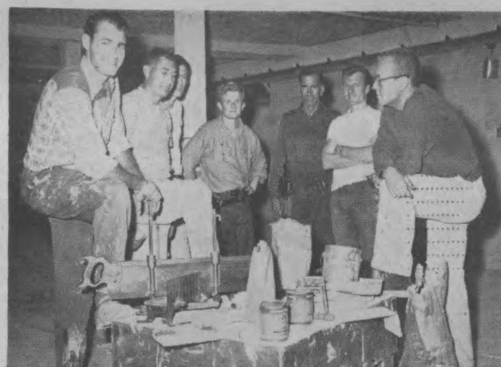
The Student Center crew pauses for the photographer. From left—Art Howard, Royce Luxton, John Johnson, two electricians, Dave Latta, and Center director Ed Allred.
