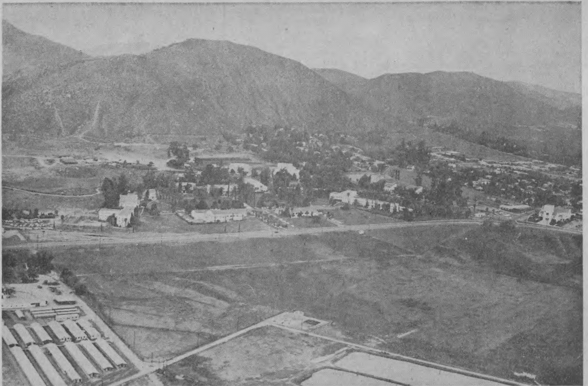
A recent aerial photo shows the campus as visiting alumni will see it. Note the new four lane highway which runs through the center of the college property. Also, at the left is the construction project of the new Calkins hall annex.
