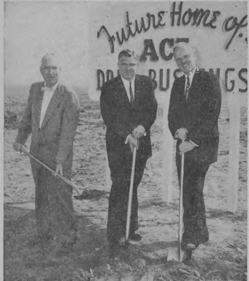
Business Manager W. E. Anderson, left, and President Norval F. Pease, right, lend a hand to President Alan A. Fisher, center, of allied Ace Drill Bushing and West Coast Aro Tool companies at groundbreaking ceremonies for the firm's new plant on LSC land. The new development will be located at the corner of Pierce avenue and Rindge road, and will employ many LSC students, managers indicate.
