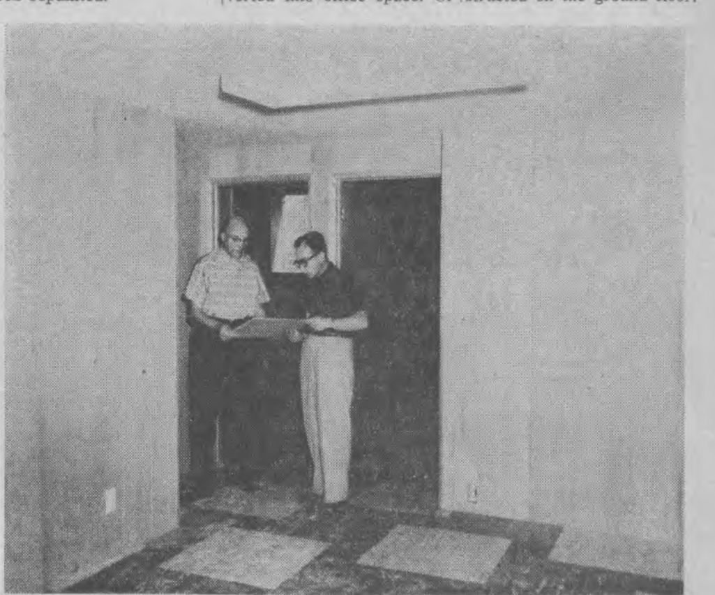
Dr. William Landeen and Prof. Fritz Guy examine blueprint of remodeling activities in lower La Sierra Hall where six new faculty offices have been provided. The offices have paneled walls and carpets on the floor.
