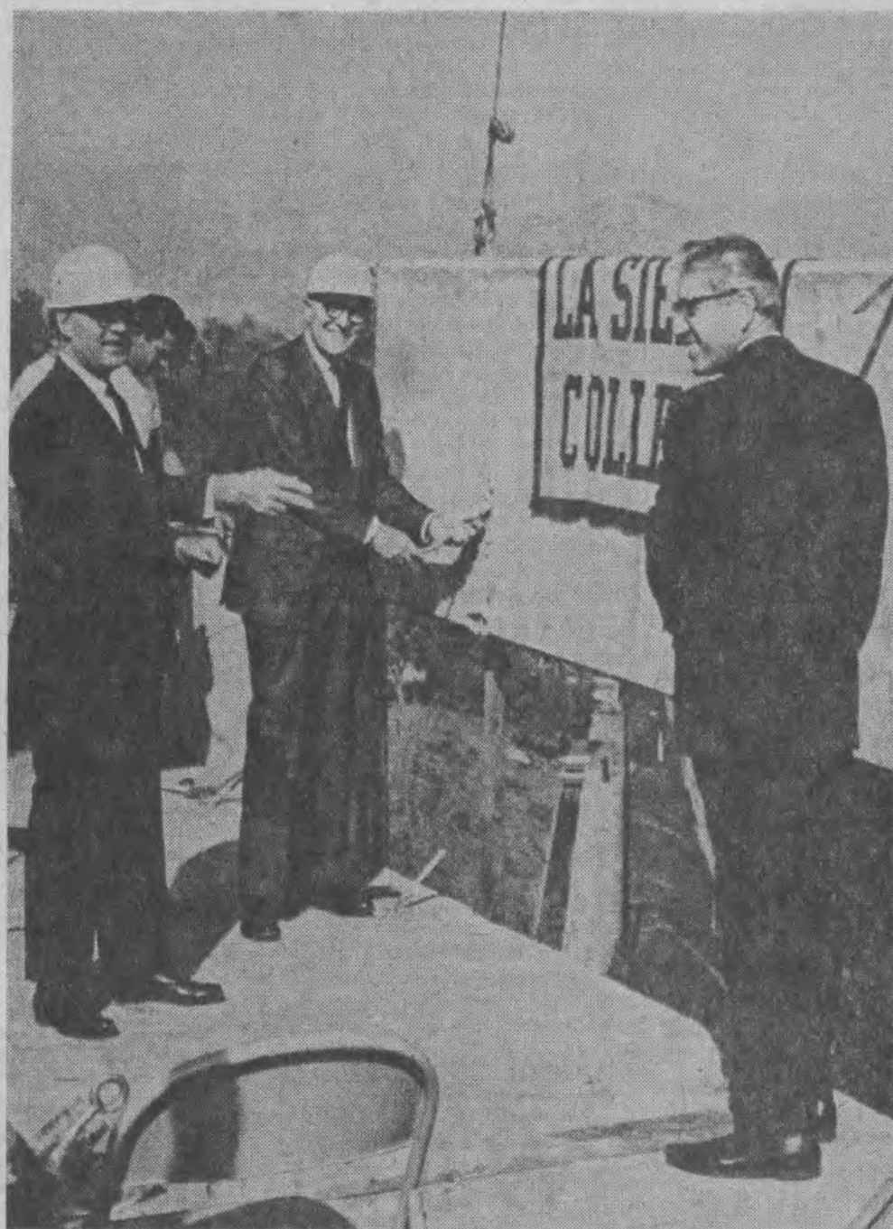
HIGH RISE COMPLETED —Ben Lewis, mayor of Riverside (center), and R. R. Bietz, chairman of the board at LSC (right), aid David J. Bieber, college president, with the placing of the last piece of concrete siding on the new men's residence hall. Topping out ceremonies were held Wednesday.
