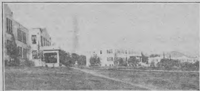
Campus from South End
