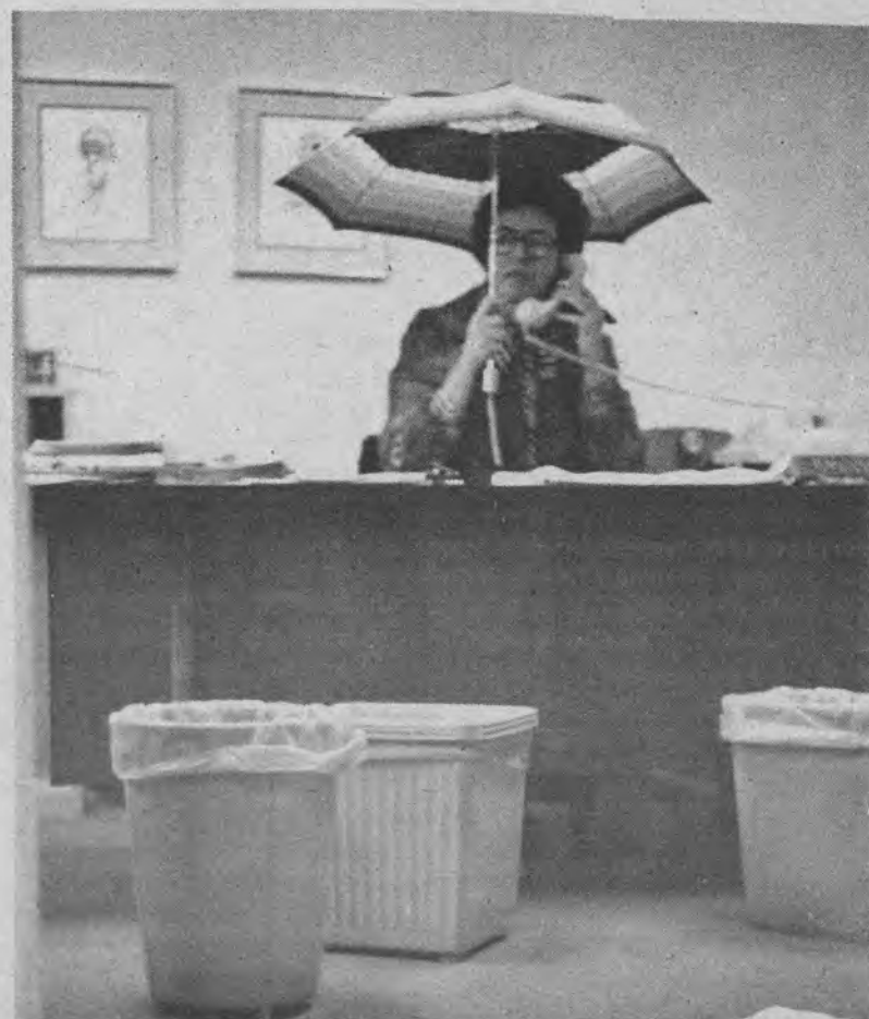
Velma Clem in the PR office tries to keep dry while she works. The roof leaked during last weeks rainstorm.
