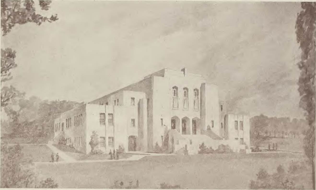
HOLE MEMORIAL AUDITORIUM. New chapel and music conservatory to be opened officially January 31, 1937. Seats 758 in main auditorium and 300 in smaller auditorium on ground floor. Also contains three music studios, ten practice rooms, eight large class rooms, offices and store rooms.
