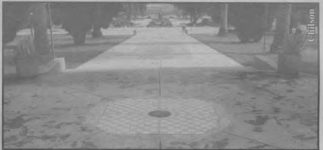
Physical plant recently replaced the concrete in front of La Sierra Hall. This small renovation is one of many scheduled to take place at LSU in the future.
