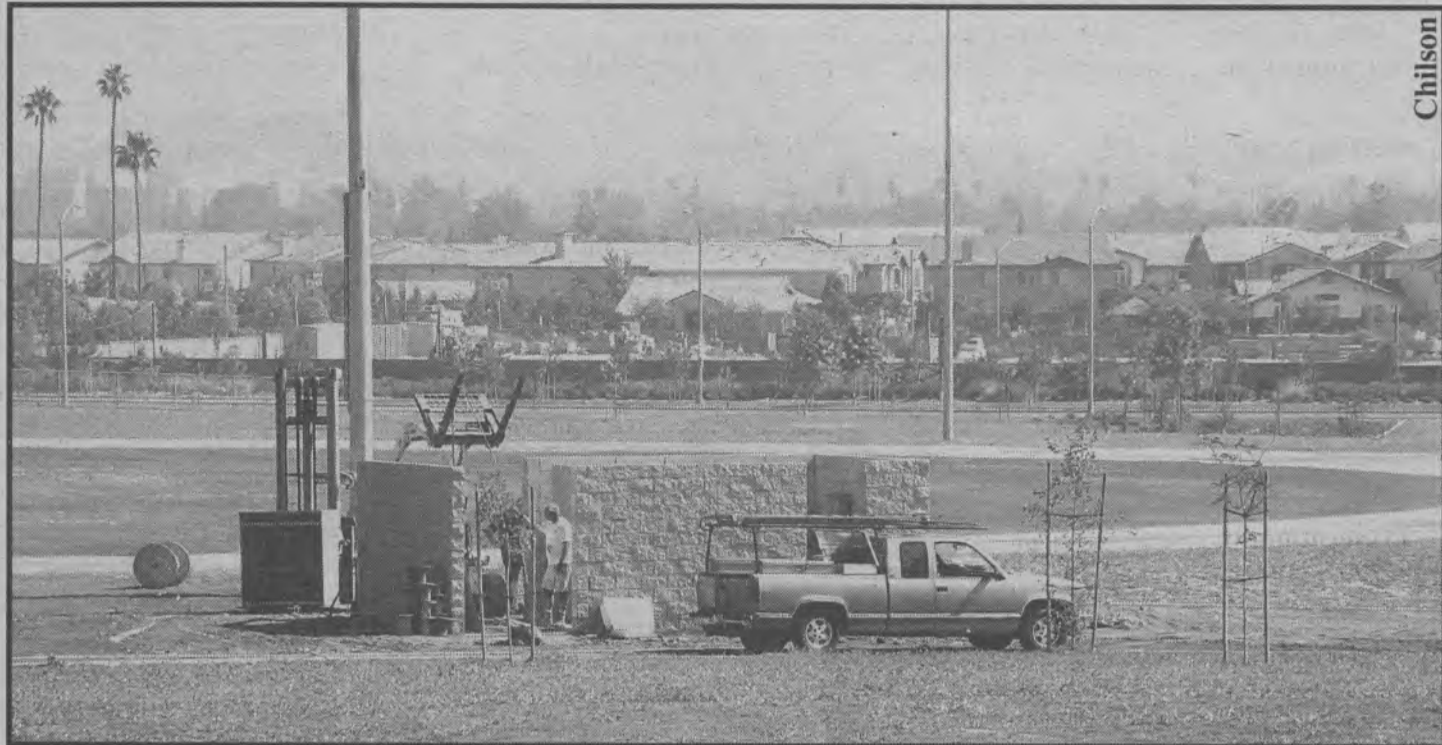
La Sierra University's athletic fields are still under construction.
